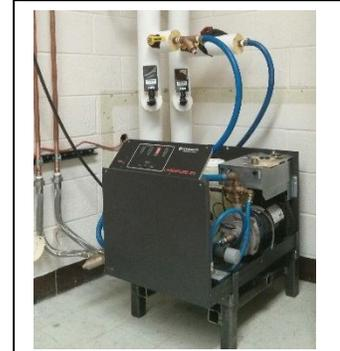
Figure 17: A Coherent LaserPure 20 chiller supplies chilled water to the Cryomech LHeP22. It is a closed-loop circulator chiller with a water pump and heat exchanger. The physics building supplied chilled water cools the heat exchanger.
