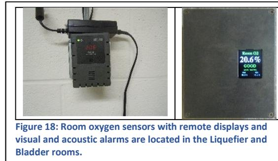
Figure 18: Room oxygen sensors with remote displays and visual and acoustic alarms are located in the Liquefier and Bladder rooms.
